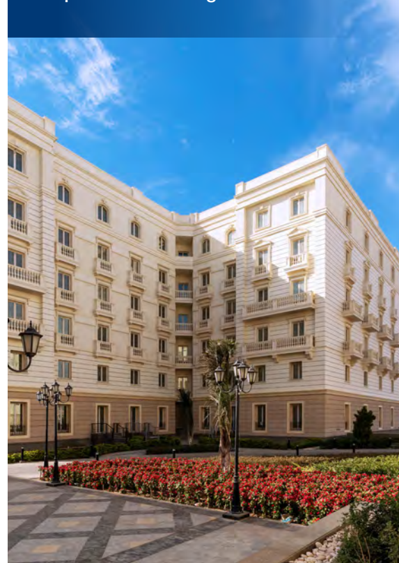
R5 Apartment Buildings
